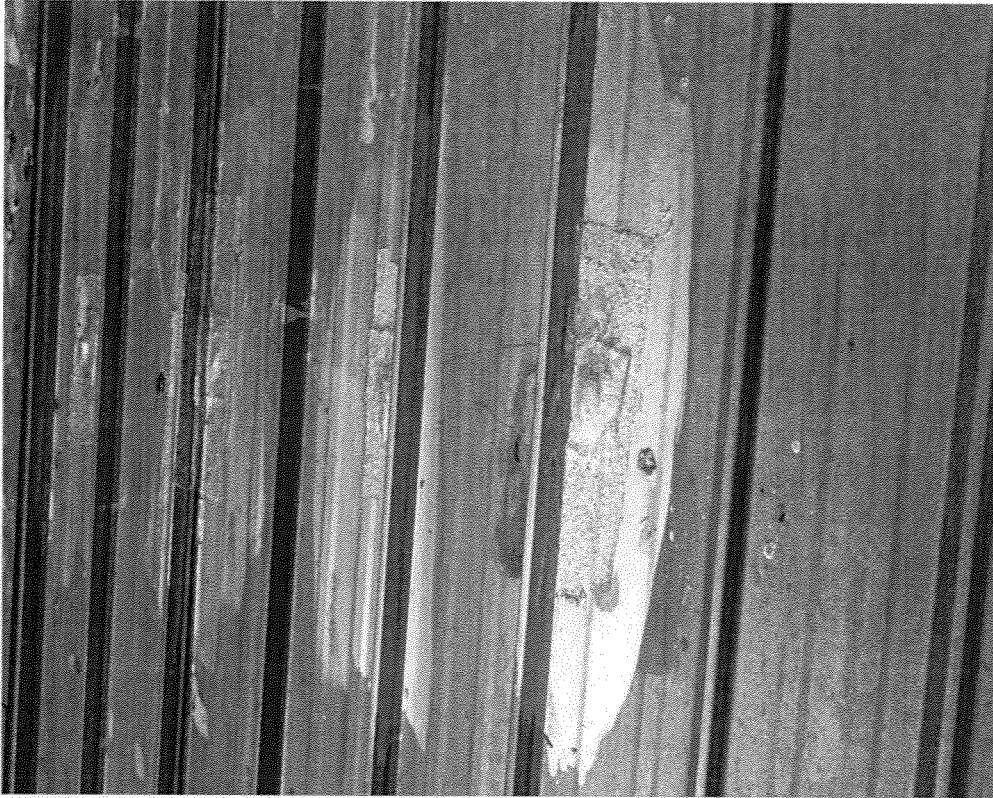
Existing roof patching
