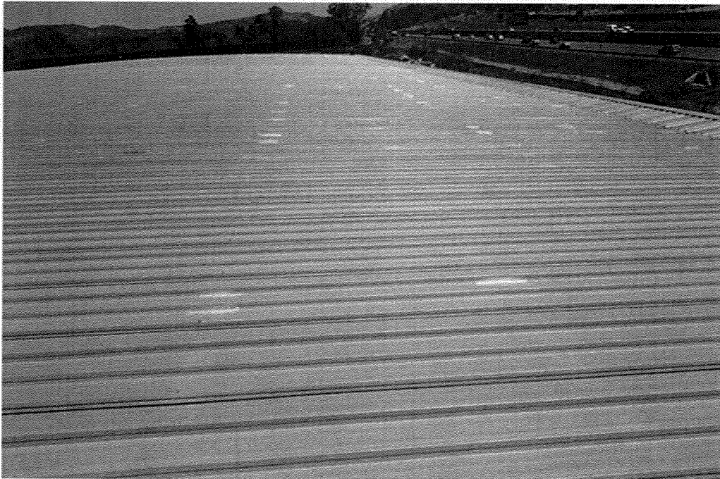
Visible silver coat paint applied over patched areas
