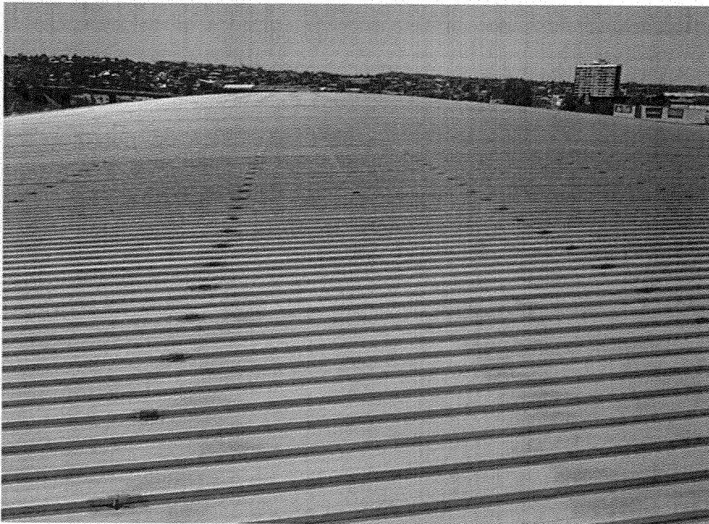
Existing Klip-lok roofing sheet at assessment building
